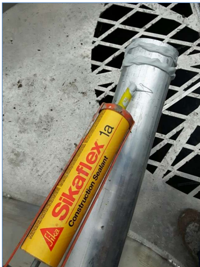
FIGURE 5 : GASKET ON OIL PIPE
